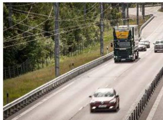
Siemens is building an overhead contact line for electrified freight transport on a ten-kilometer stretch of freeway in the German state Hesse. The first infrastructure for electric trucks line will supply electricity for the electric drive of a hybrid truck.
